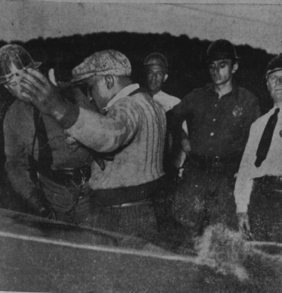
Police are pictured frisking a striking tunnel worker as he entered the area adjoining Shaft 13 of the Delaware Aqueduct project near Katonah, yesterday. All persons and cars were checked by the street guards in an effort to prevent the smuggling of dangerous weapons into the labor war.
