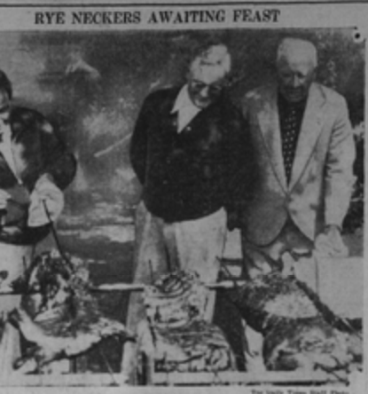
That barbeque room shows in the foreground the village above photograph in the case for the heavy ammunition, equipped on the floor of left to right, Thomas Blainey, J. S. Squire of the Village of Mamaroneck, N. Y., chairman of the Village of Mamaroneck, Republican Committee, and Richard A. Trosen, Town Chairman of the Village. Other guests were among approximately 200 persons who attended the annual barbeque of the Young Men's Republican Club of Eye Neck, held at the town hall, Sunday.
