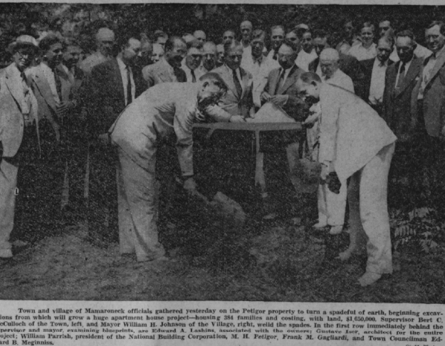
Town and village of Mamaroneck officials gathered yesterday on the Peliger project to turn a spadeful of earth, beginning excavations from which will grow a huge apartment home project—housing 284 families and costing with land, $1,000,000. Supervisor Bert C. McCulloch of the Town, left, and Mayor William H. Johnson of the Village, right, wield the spades. In the first row immediately behind the supervisors and mayor, remaining from left to right: Edward A. Lachin, president of the Peliger Building Corporation, architect for the project; William Parrish, president of the National Building Corporation, M. H. Peliger, Frank M. Gagliardi, and Town Engineer J. B. McGinnis.
