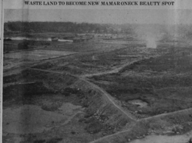
This might have been a photo of the beach-front in China, with the Great Wall in the center, but it is not—it is a picture of the area being reclaimed on Harbor Island in the Village of Mamaroneck, showing the dikes which have been completed recently.
