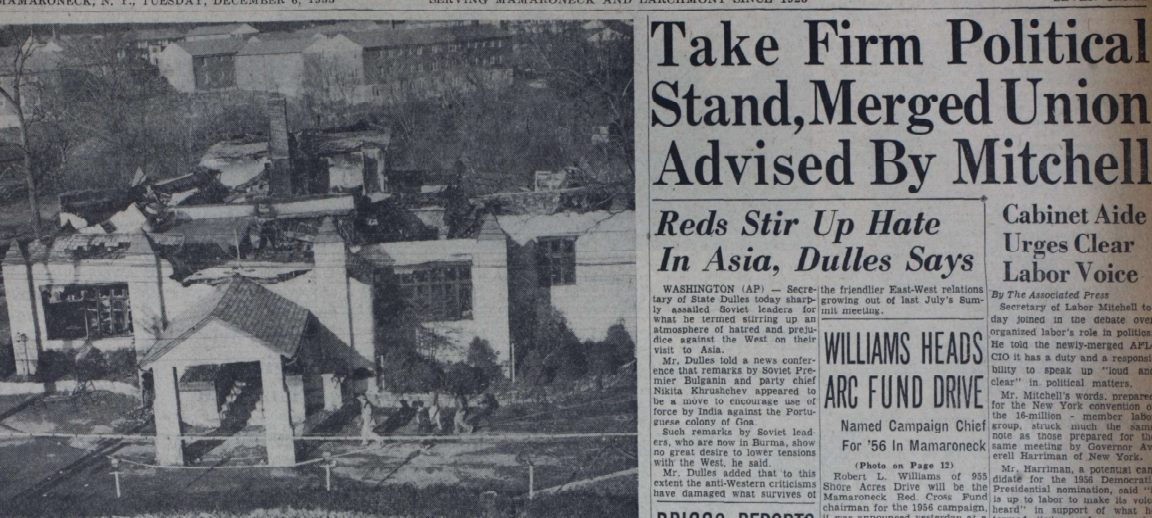
NOTHING BUT A SHELL remains of Loyal Inn, popular restaurant rendezvous on Boston Post Road, Larchmont, after Sunday night's blaze which completely gutted the building. The collapsed roof and a hint of the shambles inside the building are shown above in a picture taken yesterday. Firemen fought for more than four hours to bring the flames under control and for more than six hours before the fire was declared out. — Staff Photo by John Sarno
