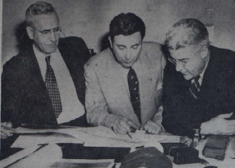
THIRTYWAY PLANNERS conferred yesterday for the first time on the actual construction of the New England Thruway which, although delayed for 30 years, is expected to get underway by mid-December, with its completion scheduled for 1953.
