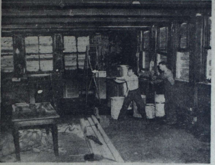
CLEANUP UP after $20,000 fire that swept through the home economics rooms in Washington Jr. High School in Mount Vernon yesterday.
