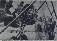
WOMEN apprentice mechanics swing a 450-horsepower airplane motor into place on an AT-9 training plane at the sub-depot of the Air Force Flying School in Lubbock. These pretty "Grease Monkeys" make efficient mechanics.
