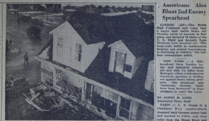
AFTER THE FLAMES WERE HEATED DOWN AND THE SMOKE CLEARED AWAY THE ABOVE SCENE EMERGED AS PART OF THE WRECKAGE FROM LARCHMONT'S WORST FIRE IN 22 YEARS SATURDAY AFTERNOON ON PALMER AVENUE. THE BLAZE, SAID TO HAVE STARTED IN A DEFECTIVE FLUE, SPREAD THROUGH SIX STORES AND ROUTED FOUR FAMILIES FROM THE SECOND STORY APARTMENTS BEFORE IT WAS BROUGHT UNDER CONTROL BY THE FIRE DEPARTMENT'S LARCHMONT, THE TOWN OF MAMARONECK AND NEW ROCHELLE. THE LOWER PHOTO SHOWS THE DEPUTY CHIEF JOHN HAYCOCK POINTING TO THE CHARRED RAFTERS UNDER ONE OF THE ROOFS. THE DAMAGE HAS BEEN ESTIMATED BY MUNICIPAL OFFICIALS AT VARIOUS FIGURES FROM $12,000 TO $25,000.
