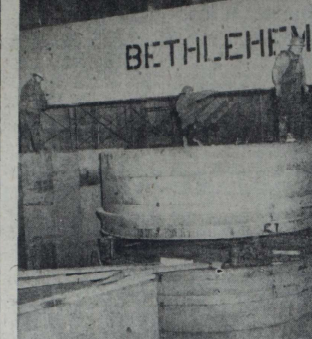
GENERAL VIEW OF THE 2500 foot cyclotron which Columbia University has installed in its new nuclear research center at Nevis, Irvington. Workmen to which is a key part of the cyclotron which is the largest, most powerful cyclotron ever built—38 blocks of steel, each weighing 60 tons.
