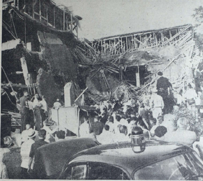
THIS SCENE OF DESTRUCTION resulted in Scarsdale late yesterday afternoon when a four-story superstructure of a new office building collapsed as workers were pouring the last batch of concrete on the roof. Ten survivors were dug out of the twisted ruins—some of them hours after the disaster which mobilized Civil Defense and other rescue squads from Scarsdale and neighboring communities. Three workers were killed in what District Attorney Samuel Paley described as "the worst building disaster I have ever seen in what District 'Westchester'."
