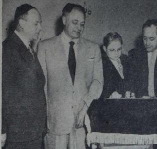
FIRST CONTRACT for the construction of the new Westchester Jewish Center at Rockland and Palmer Avenues, Mamaroneck, was signed last night by Hyman L. Pederman, president of the congregation...
