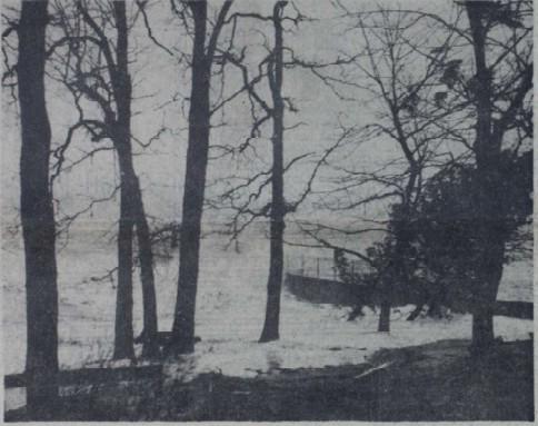
THE BREAKWATER at the foot of Rushmore Avenue, Mamaroneck, usually standing well above high water, is almost submerged in the photo above as the wind-blown tide neared its peak Saturday. The picture was taken from the porch of a home, and above the water gushing up on the lawn to the street.
