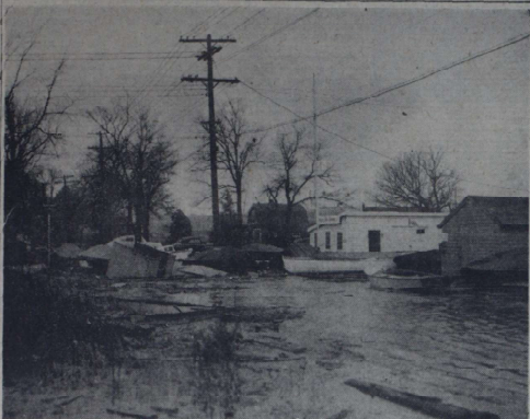
WRECKAGE of boats and buildings was strewn haphazardly Saturday as Rushmore and Seneca Avenues by the wild wind and wider tide of the gale. The boat pictured above was driven onto Rushmore Avenue near McMichael's Boat Yard.
