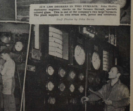
GADGETS GALORE in the plant's boiler room keep Engineer Foster busy. This automatic control board is the pulse of the plant which last year melted nearly 100,000 tons of raw sugar and produced approximately 25,000 tons of dry sugar and 125,000 tons of liquid sugar.
