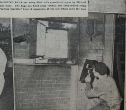
IT'S 1,800 DEGREES IN THIS FURNACE. John Foster, stationary engineer, checks on the furnace through specially colored glass. This is one of the company's two large furnaces. The plant supplies its own steam heat, power and electricity.
