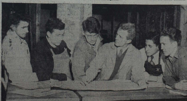
IN FRONT OF THE FRAME STRUCTURE on which they get practical training construction lab students work over a blueprint for new details. The building, shown behind them, includes all construction problems, featuring a bay window, main stair well and similar problems. Left to right are Robert Cudney, Woodlawn; George Phelps, Yve; John Mowry, White Plains; William Britt, assistant professor; Frank Paradise, Port Chester; and Nathan Pierdubica, Yonkers. Before proceeding with a new set-up in the construction, the students will map in detail the work to be accomplished and methods to be used.
