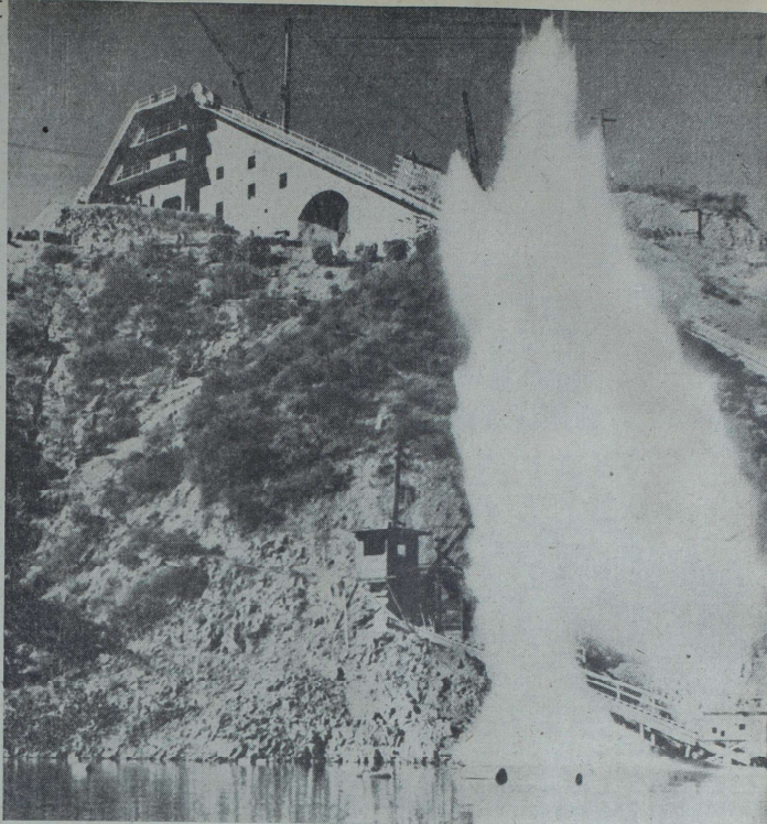
A geyser is hurled into the air as a 2,000-pound torpedo rips into the water. On bluff is part of variable angle launcher being built.
