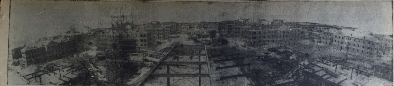
PANORAMA VIEW shows the 31 buildings of Franklin Delano Roosevelt Veterans Hospital at Cruisers Point, near Peekskill, under various stages of construction. The $2,400,000 project on 283 acres of the former County-owned Cruisers Park will have a capacity of 1,084 beds. Work on the buildings
